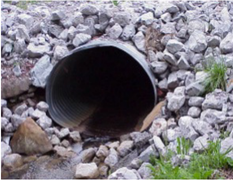
Figure 9. Riprap to stabilize outlet
