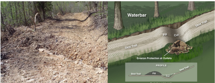
Figure 7a. Water bar construction
